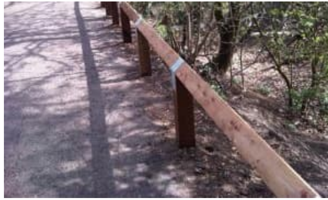
Figure 21. Example Birdsmouth Fencing (sawmill timber)
